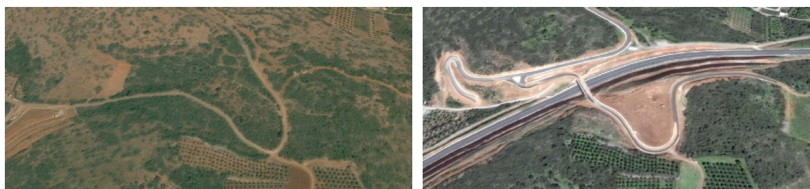
Figure 1: Terrain before (left) and after the construction (right).
